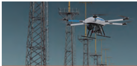
电力巡检 / Power inspection
